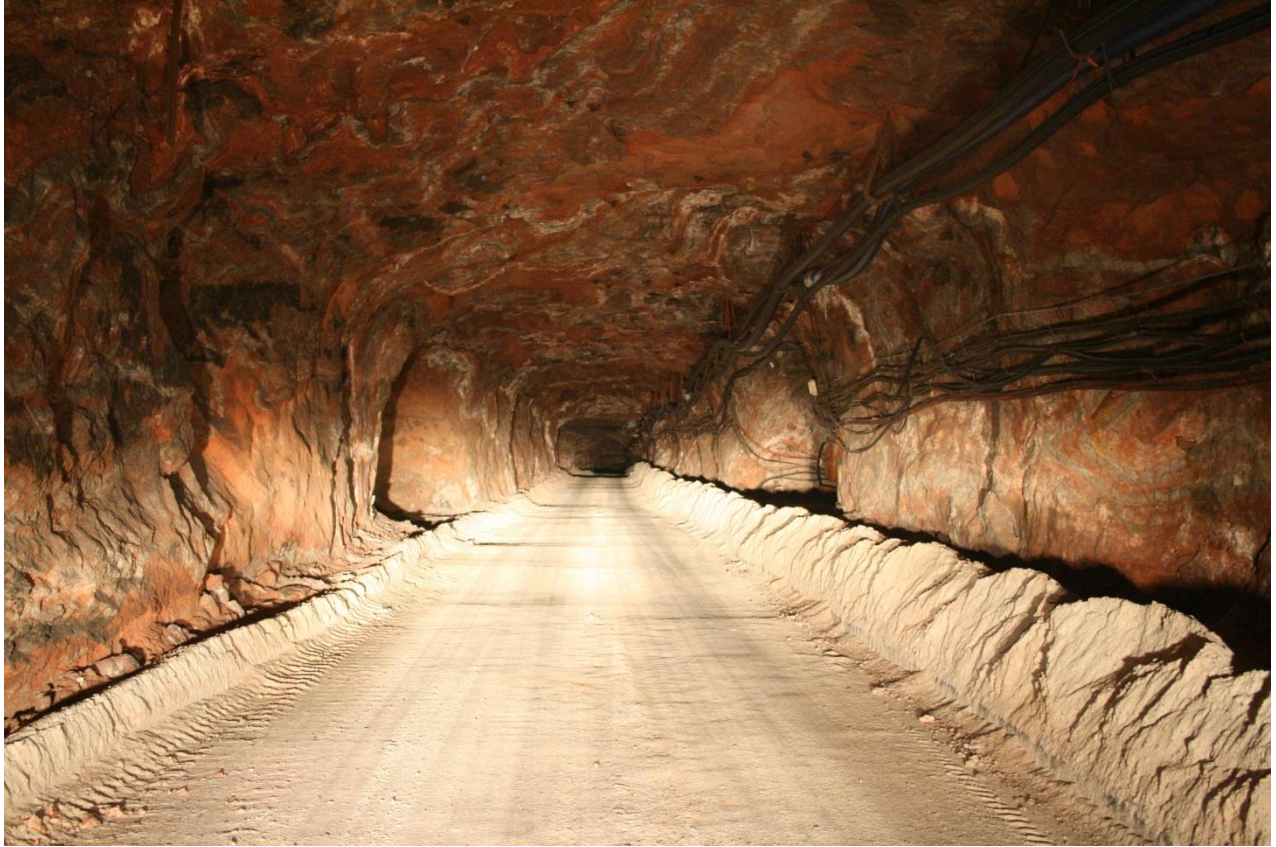
figure 2: main roadway with sensor cables for the post-shutdown operation and their covering with salt on the floor on both sides
