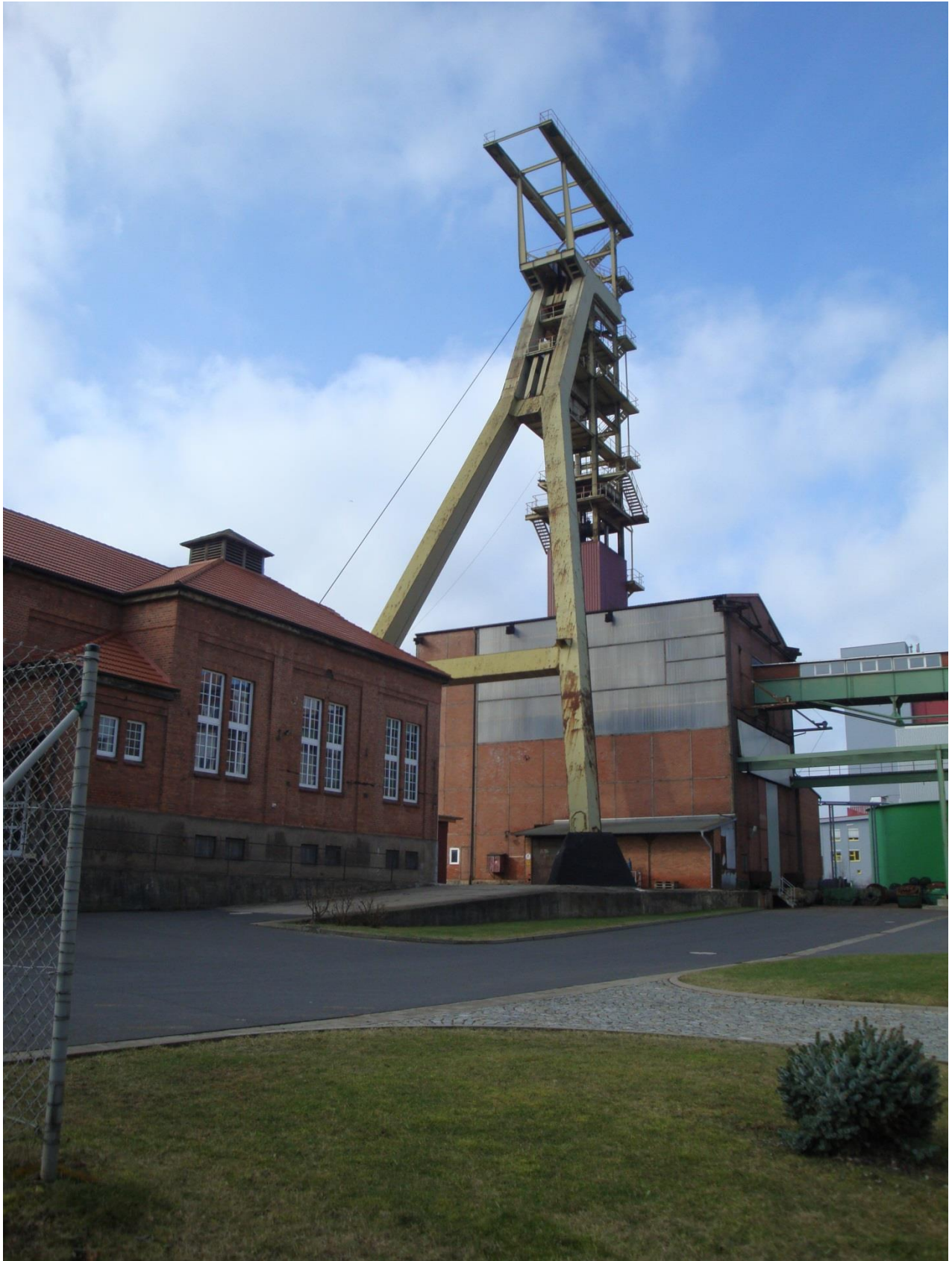
figure 1: shaft tower shaft II with hauling engine
